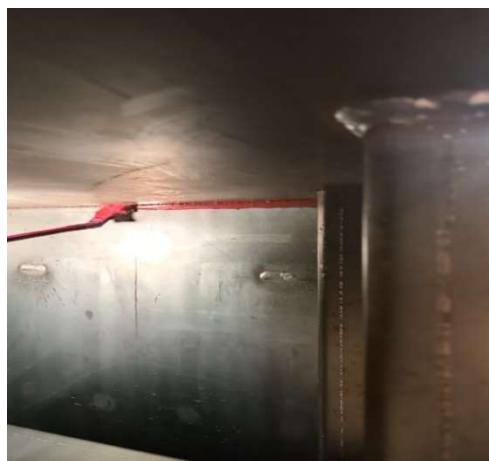
Figure 13. Application of the penetrant to the internal impermeable welds
