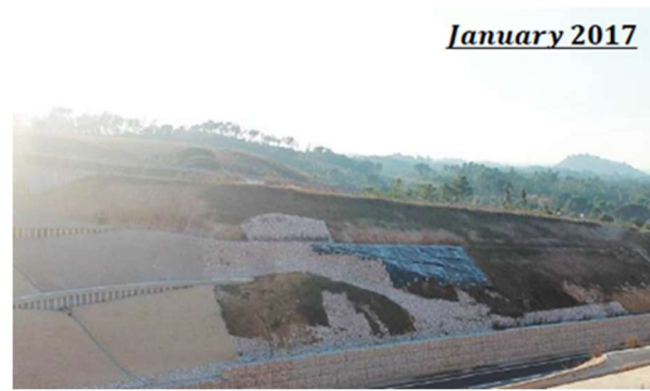
Figure 8. View of slope after interventions [11].
