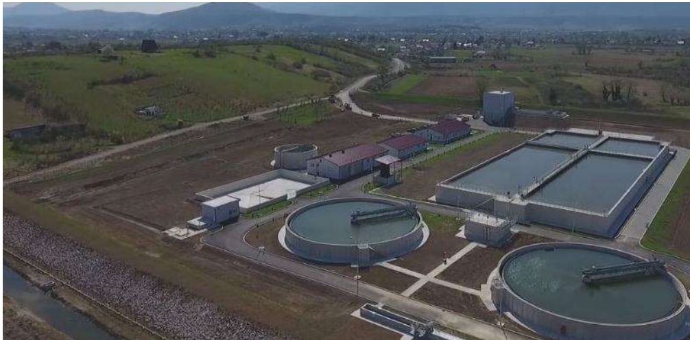
Figure 2. Wastewater plant in Bihać [5].
