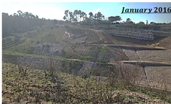
Figure 7. Construction of walls made of metal piles [11].
