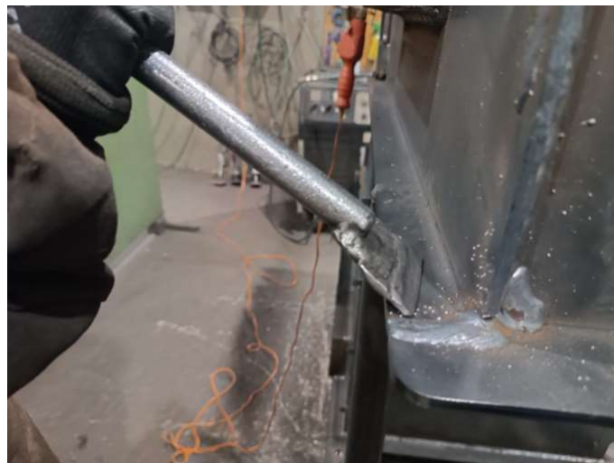
Figure 11. Surface cleaning with a steel brush
