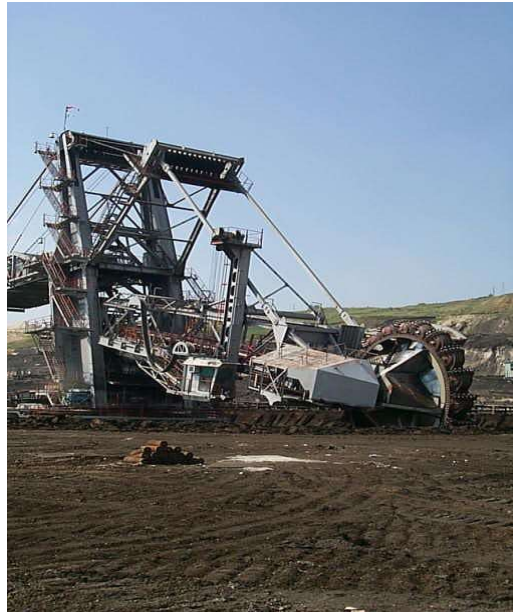
Figure 1. Rotary excavator SH 630 before overhaul.
