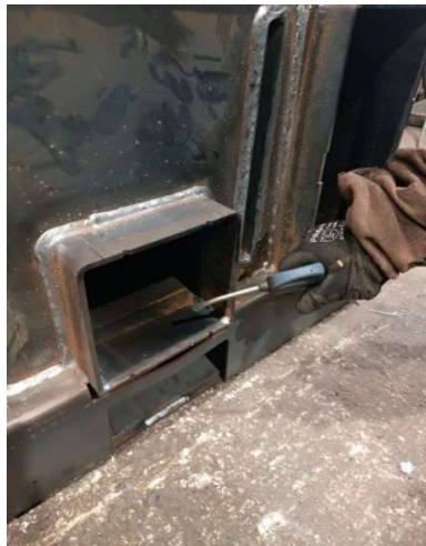
Figure 12. Surface cleaning with compressed air
